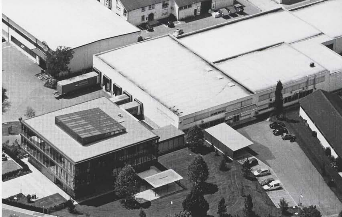
Administration Building and Production Building, Weingarten (DE)
